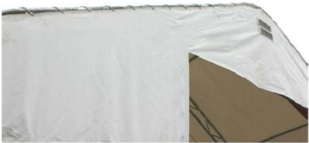
Figure 1: Tarp corner detail
