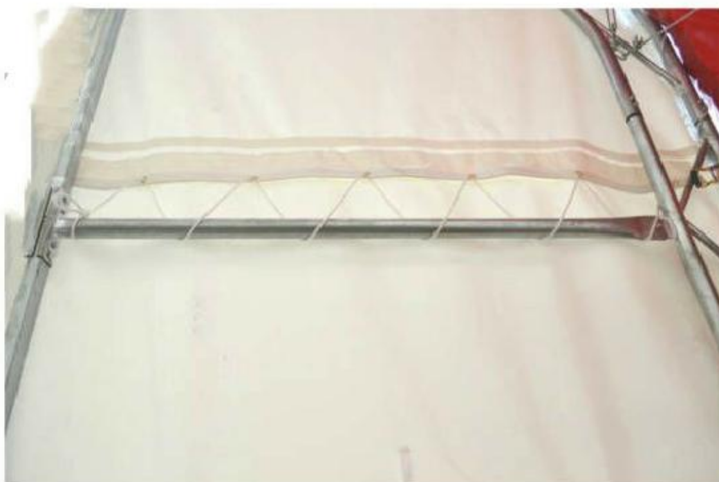
Figure 2: Interior view of the tent structure.
