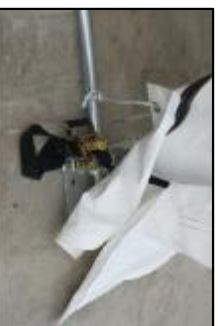
Figure 11 Fastening the two ends of the Roof Cover
