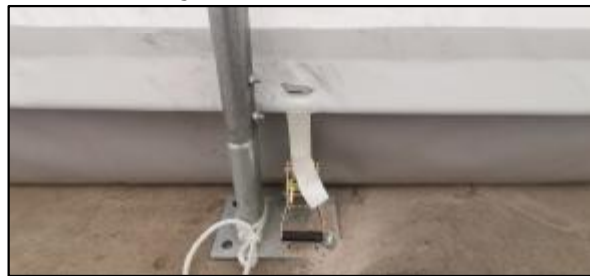
Figure8: Pull the Roof Cover over the frame evenly
