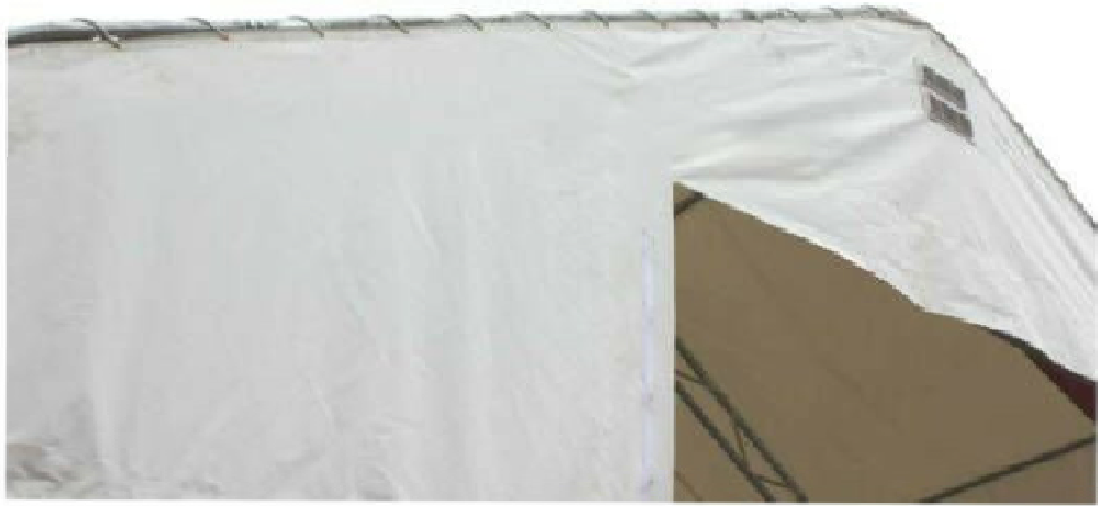
Figure 11: Tarp covering the structure
